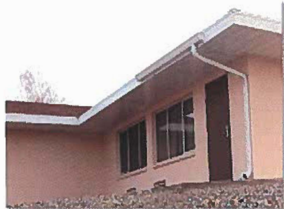
Photo 6-9. Classroom doors and windows
