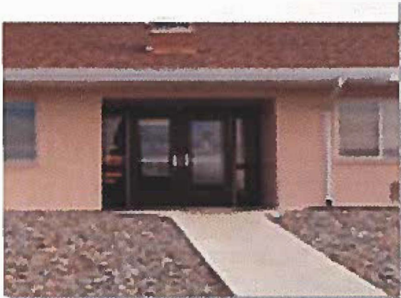
Photo 6-8. Doors to unfenced area
