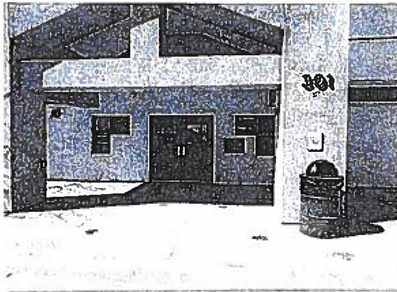
Photo 6-1. Hawthorne Elementary School Front Entrance Leading to Office
